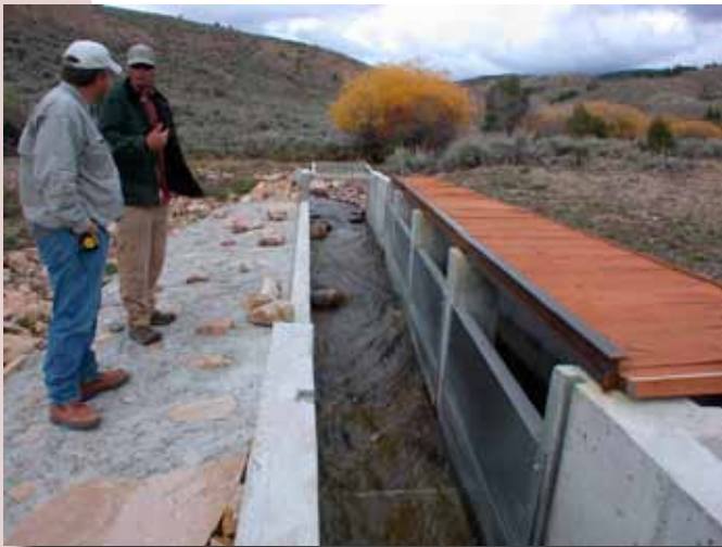
One of the simplest possible fish screens: a vertical screen cleaned by rapid flow in the concrete channel at left. Water passes through screen in center and is transported to a pivot irrigation system. Grade Cr, tributary of Bear River, Wyoming. Adult fish migrating upstream to spawn do pass this screening system with the help of rocks placed on the concrete floor.
