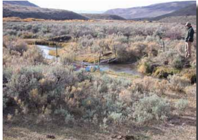
A downstream view of a typical pole-and-tarp diversion in western Wyoming. The open diversion channel exits to the right.
